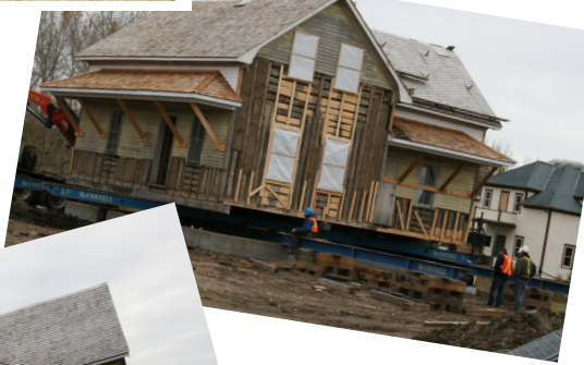
The house placed on the foundation
